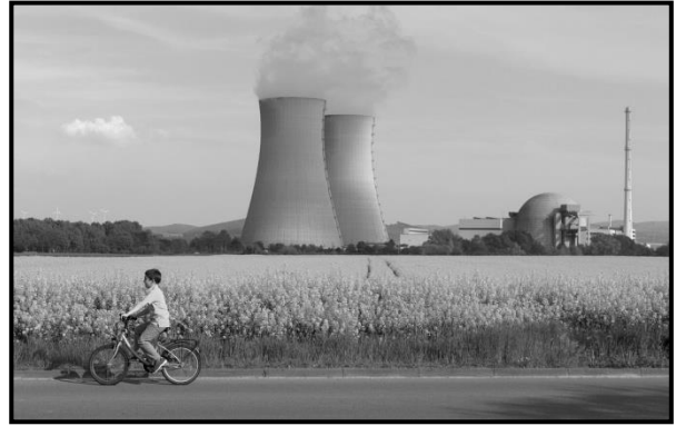
Nuclear power station
